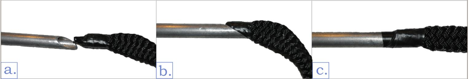
Insert the rope with the needle into the tube and place it around the cabled trunk. **a.** Pull about 60 to 70 centimetres **b.** of the rope from the tube, measuring the length from the splice in such a way that the individual parts of the rope that encircles the tree will be kept an angle of less than 45° at the first splice. **c.**
